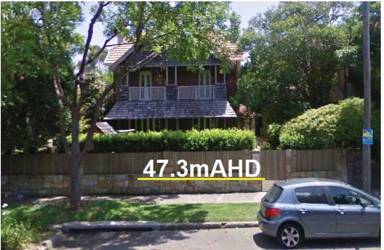
Lang Road, Centennial Park, showing approximate elevation of peak flood levels during a 2Y ARI storm event.
